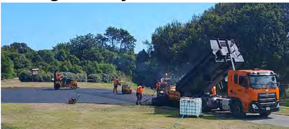
Graeme of Rocka Excavation captured McCormack Asphalt's laying of the top coat.
