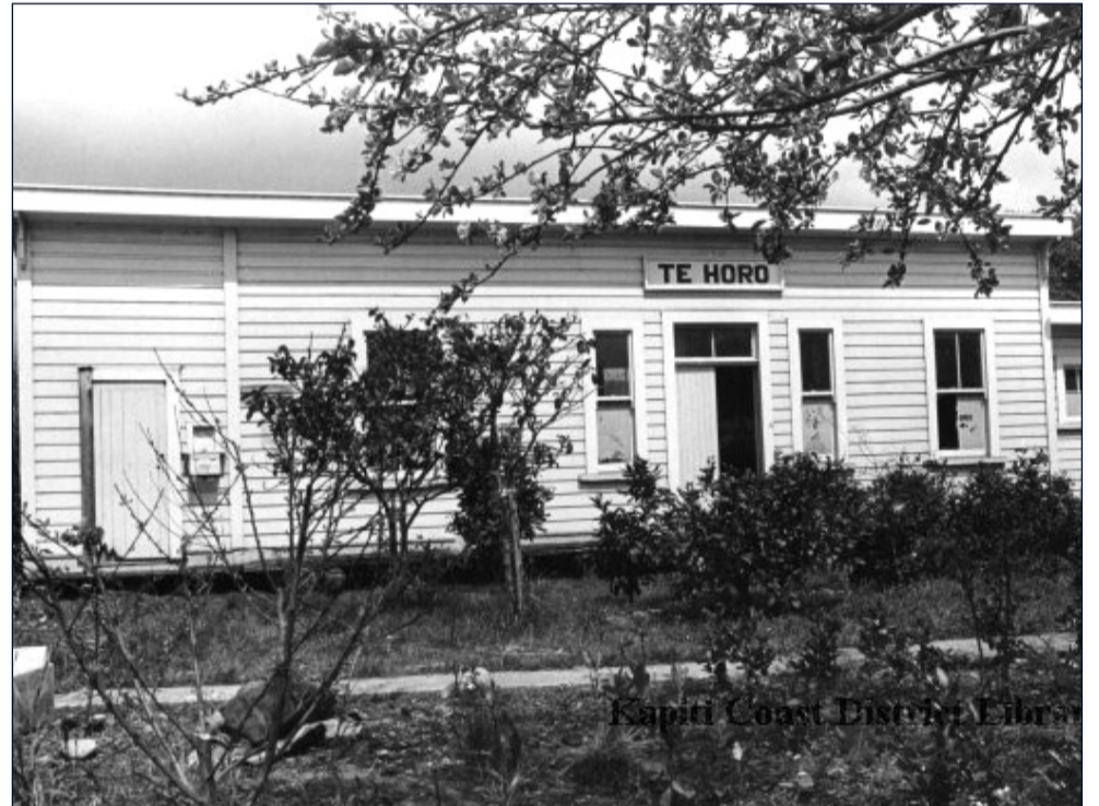
Te Horo Railway Station, 1979. Image courtesy of Kāpiti Coast District Council Archives
